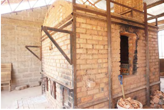
Figure 3-22 The kiln in PHW
