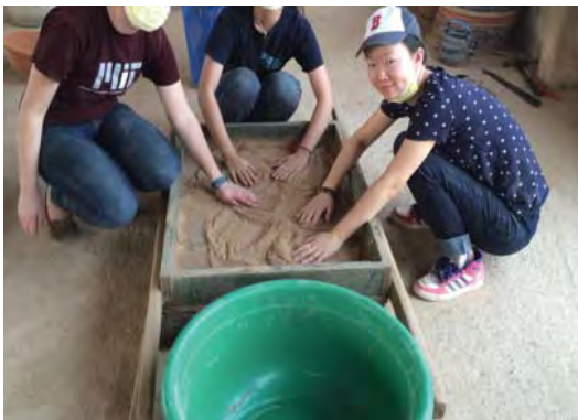
Figure 3-14 Sieve the rice husks by hand
