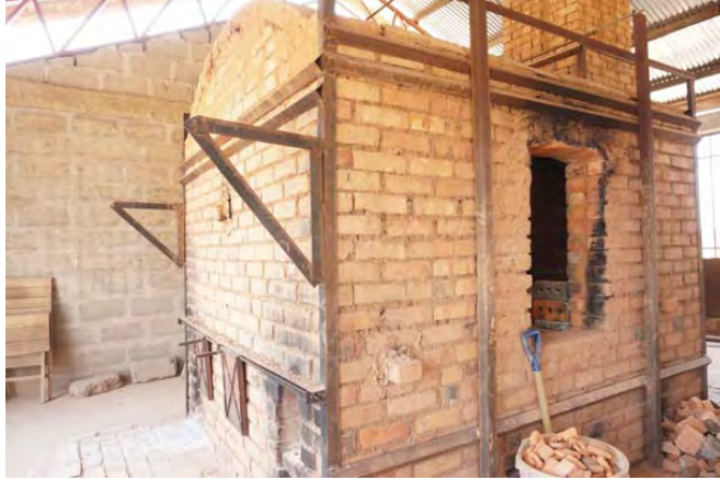
Figure 3-8 The kiln in PHW
